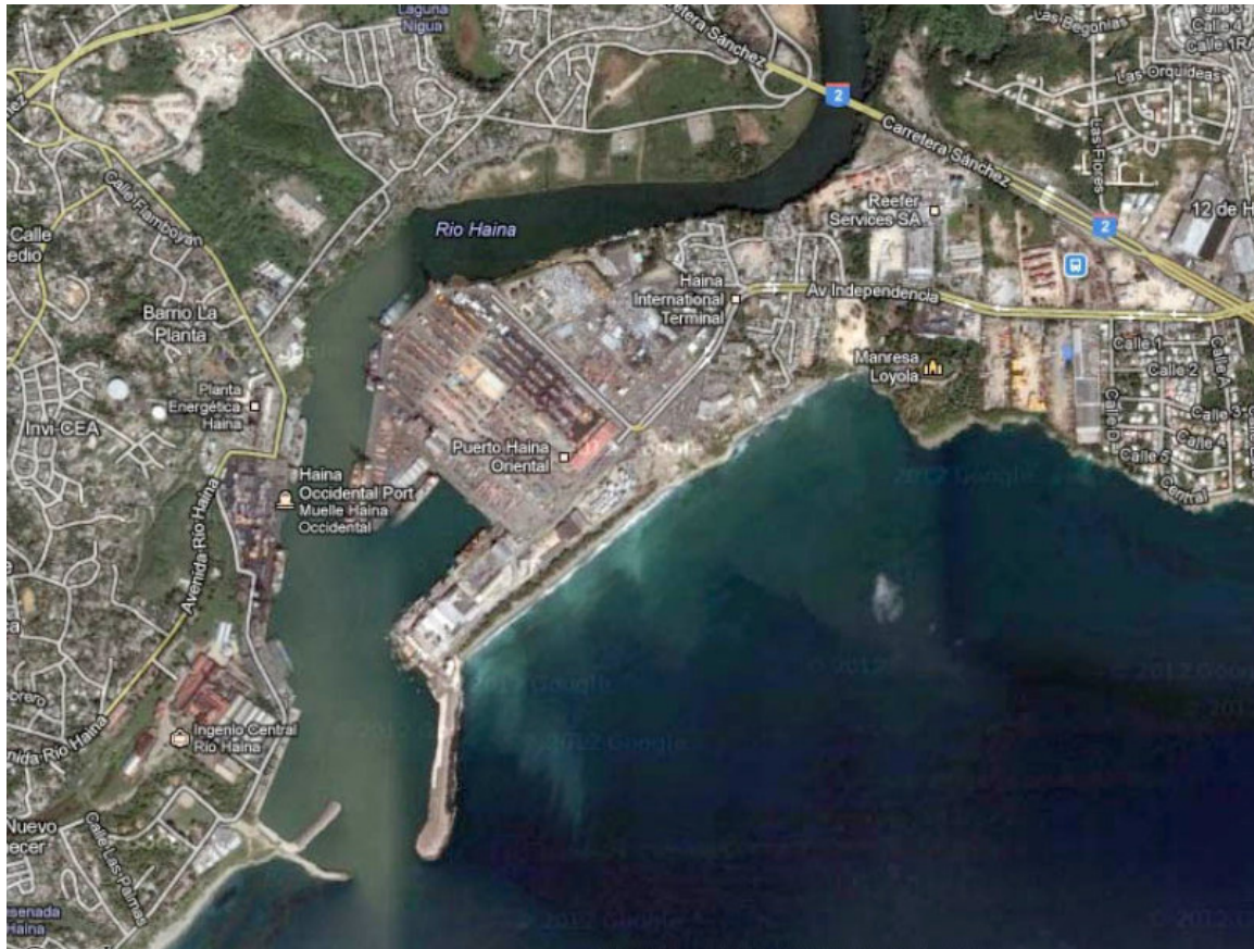
Figure 20. Puerto de Haina
